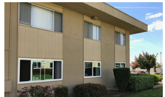
Comparison of old windows vs. new dual-pane windows at North Park Apartments in Oildale, CA.
